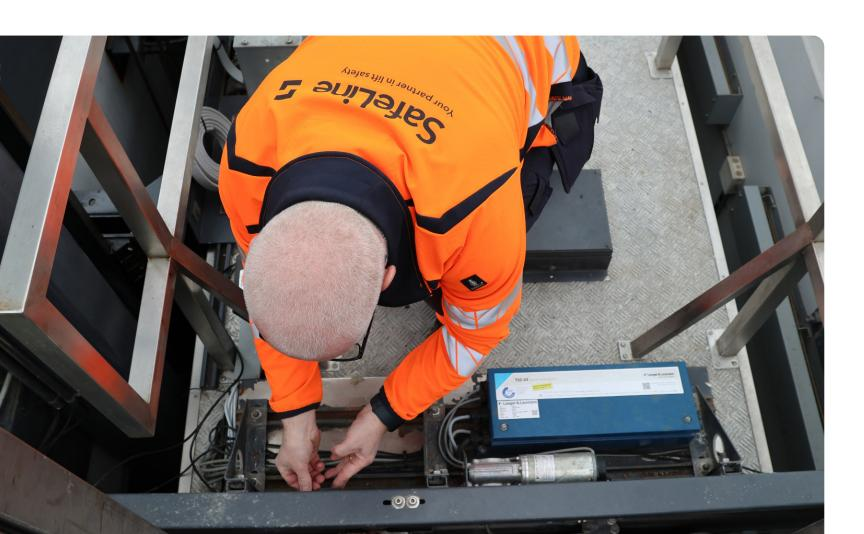
Install the LYRA on the car roof and connect LYRA to the USB door sensor.
